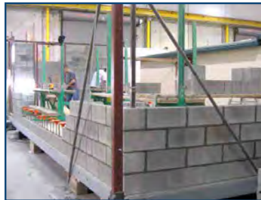
5 | CMU Walls Constructed on Concrete Slab
