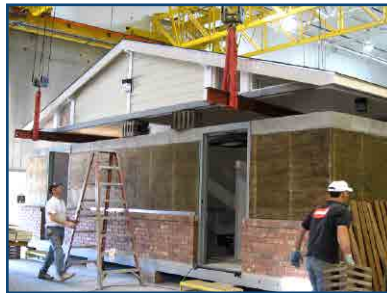
7 | Roof is Installed on CMU Walls
