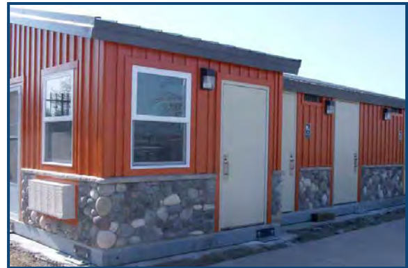
Laundry Room + Restrooms
