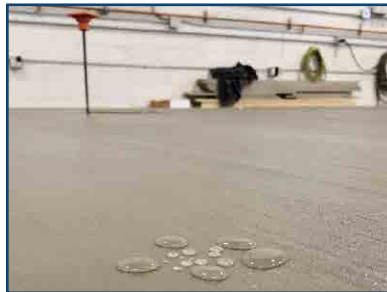
4 | Finished Slab of Specialized Moisture Resistant Concrete
