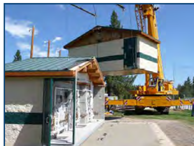
10 | Drop-In-Place Installation with a Crane
