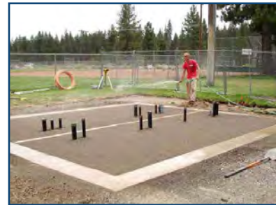
9 | Sub-Grade Pad Preparation
