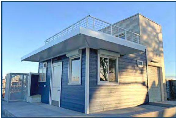
Lifeguard Station | Shower & Restrooms
